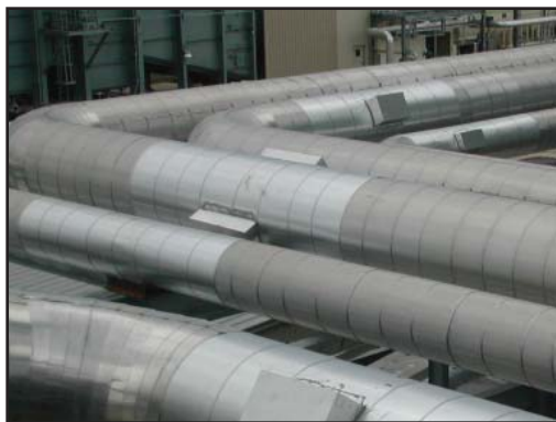
*Steam lines after installation of PT&P's newly designed shoes
