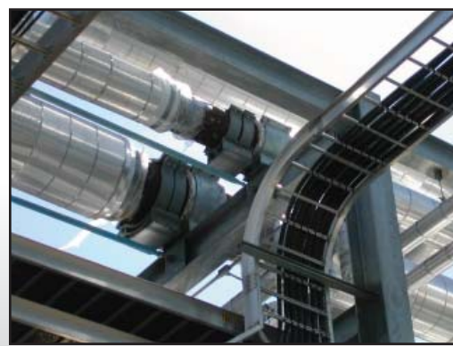
*Removal of defective supports and installation of new shoes
