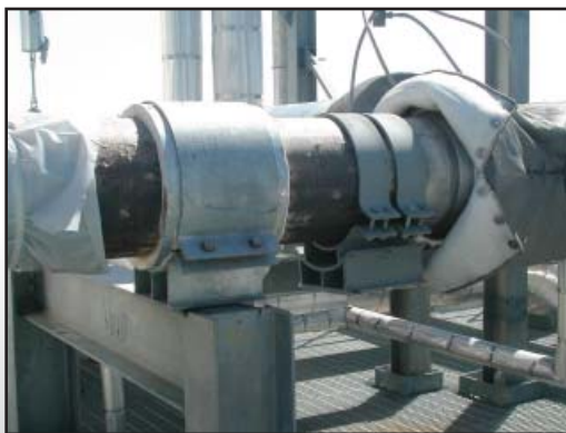
*Removal of defective supports and installation of new shoes
