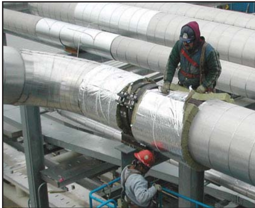
*Restoration of insulation
