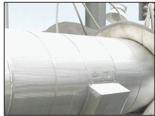
*Steam lines after installation of PT&P's newly designed shoes
